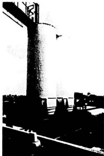
A view of the new gravity loading bins. The state capitol can be seen in the far right background.
